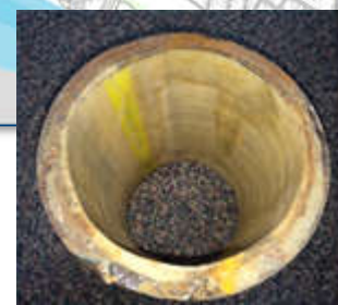
Cast Iron Watermain - After Relining
