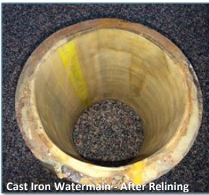
Cast Iron Watermain - After Relining
