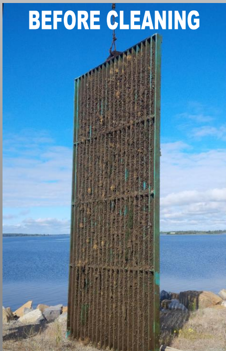
The raw water intake screen is removed for its annual cleaning and inspection on September 12 th , 2018.
