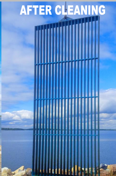
The raw water intake screen is removed for its annual cleaning and inspection on September 12 th , 2018.
