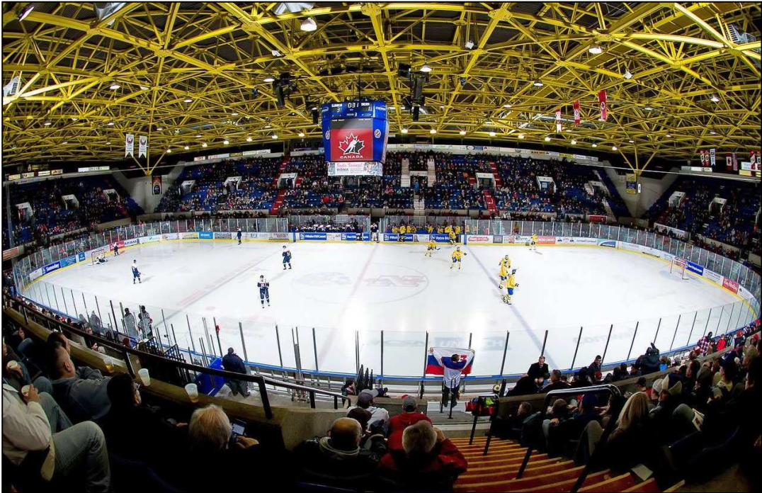
The photo above shows the existing arena lighting at the Ed Lumley Arena. There is additional lighting around the perimeter that is used for high profile games (such as the IIHF game shown). These additional fixtures aren't used during regular programming as they generate too much heat and impact ice quality if left on for long durations.
