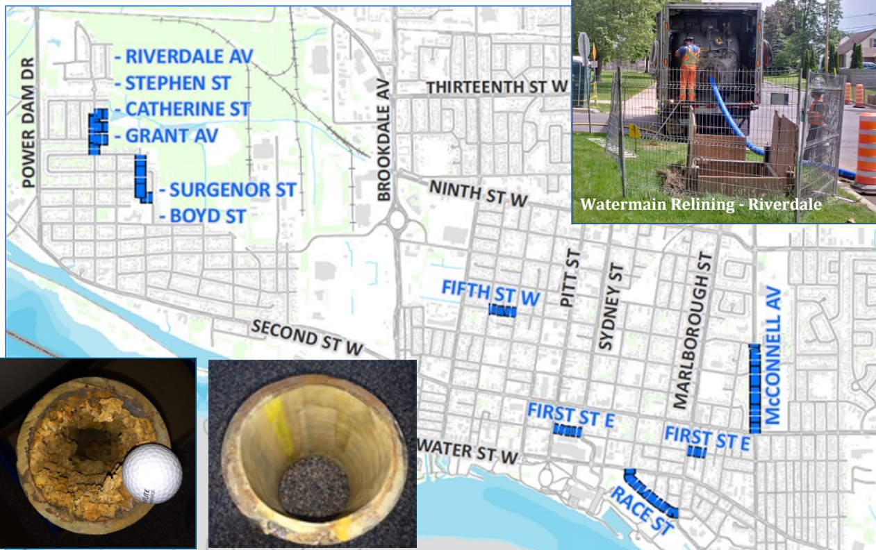
Cast Iron Watermain Before Relining
