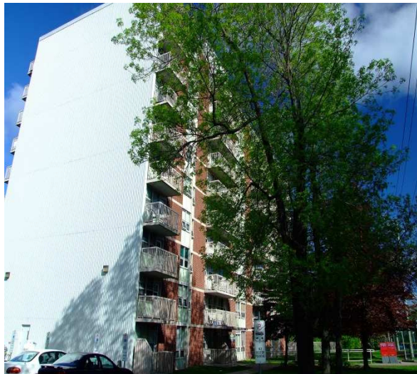
540 Adolphus, 105 Senior Units, Cornwall
