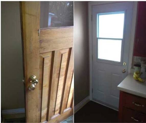
Before and after picture of a door replacement
