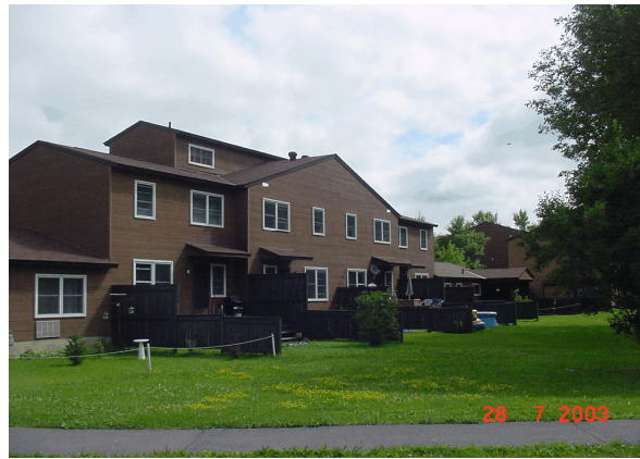
Royal Oaks Co-Operative, 70 Family Units, Cornwall
