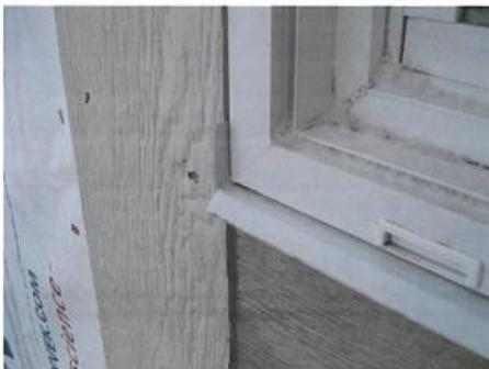
Sill Flashing with End Dams
