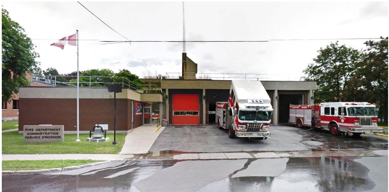
Figure 5: Existing Fire Station 1 Headquarters Located on Fourth Street West (Ground View)
