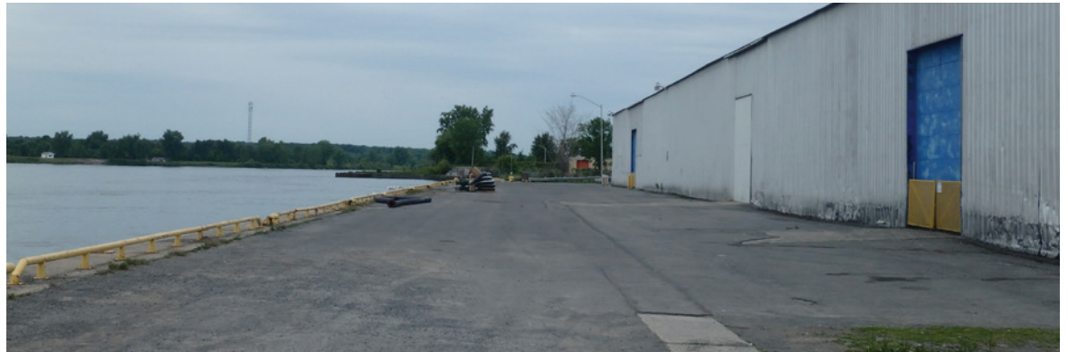
figure 32. Aging Infrastructure with restoration potential
