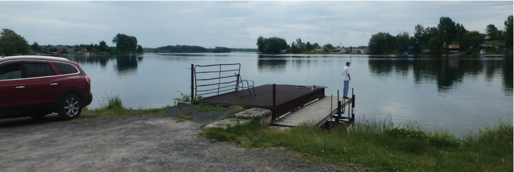
figure 68. E.7 Boundary Road Boat Launch (Before)
