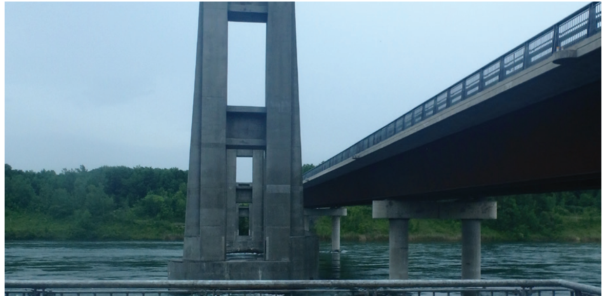
figure 19. Brookdale Avenue Bridge
