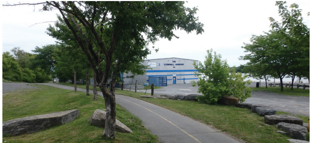
figure 28. View of Cornwall Harbour
