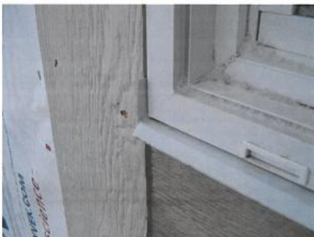
Sill Flashing with End Dams
